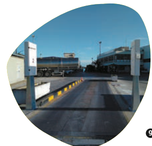
Saphygate zone exit gantry
